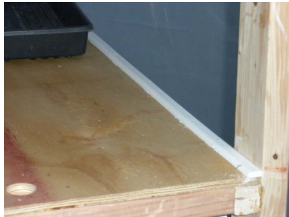
Figure 10. Shoe molding installation complete
