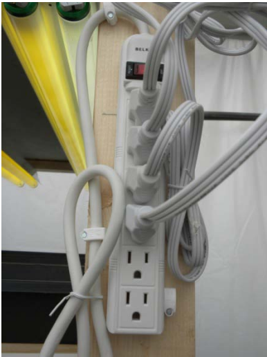
Figure 11. Electrical power cords routed to minimize accidental unplugging
