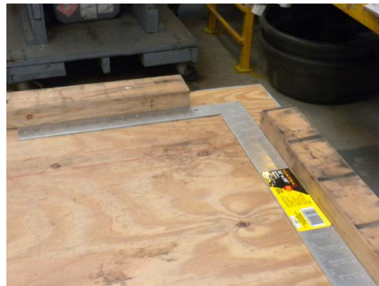
Figure 2. Creating a jig to assure square corners
