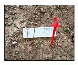
Metal wire staple on the left and the plastic staple on the right. These are used to secure covering material.
