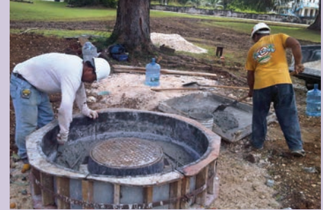
EPA has funded sewer improvements on Saipan.
