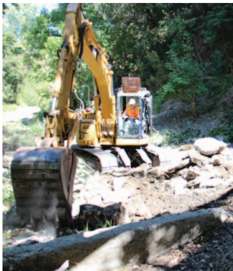
Workers remove a barrier to fish migration in San Francisquito Creek.
