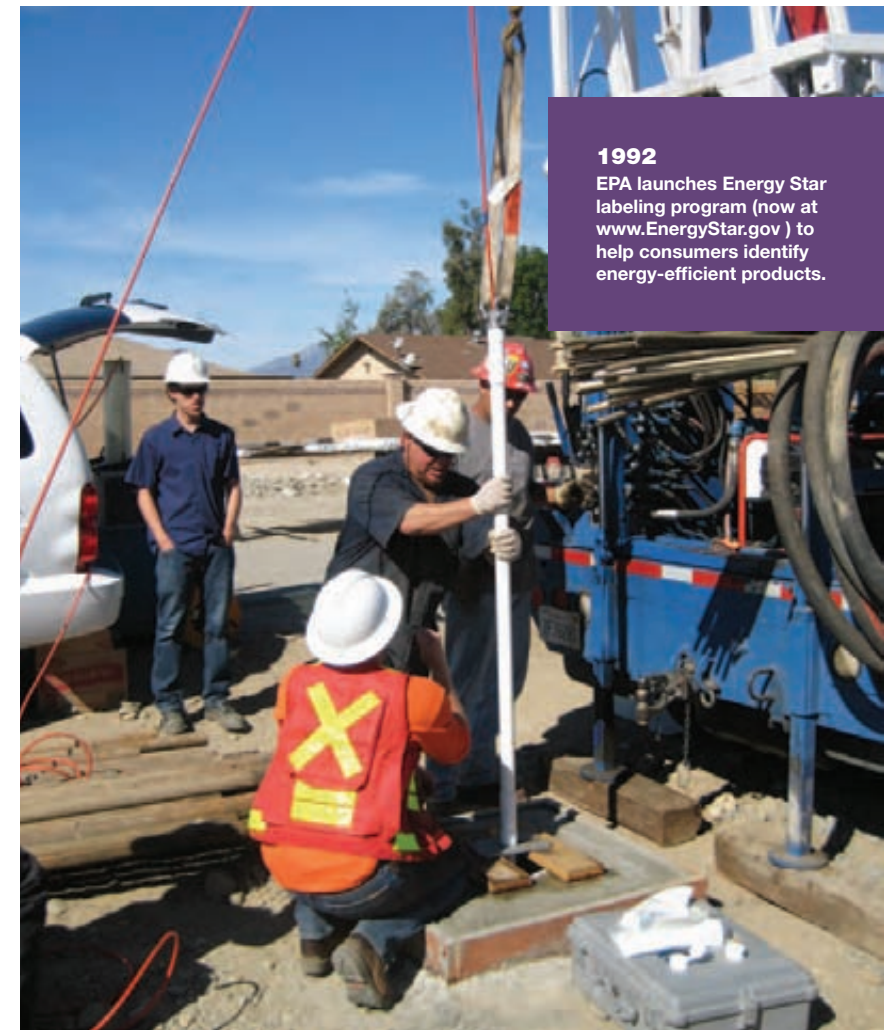
Right: EPA contractors constructing a groundwater monitoring well at B.F. Goodrich Superfund Site.
