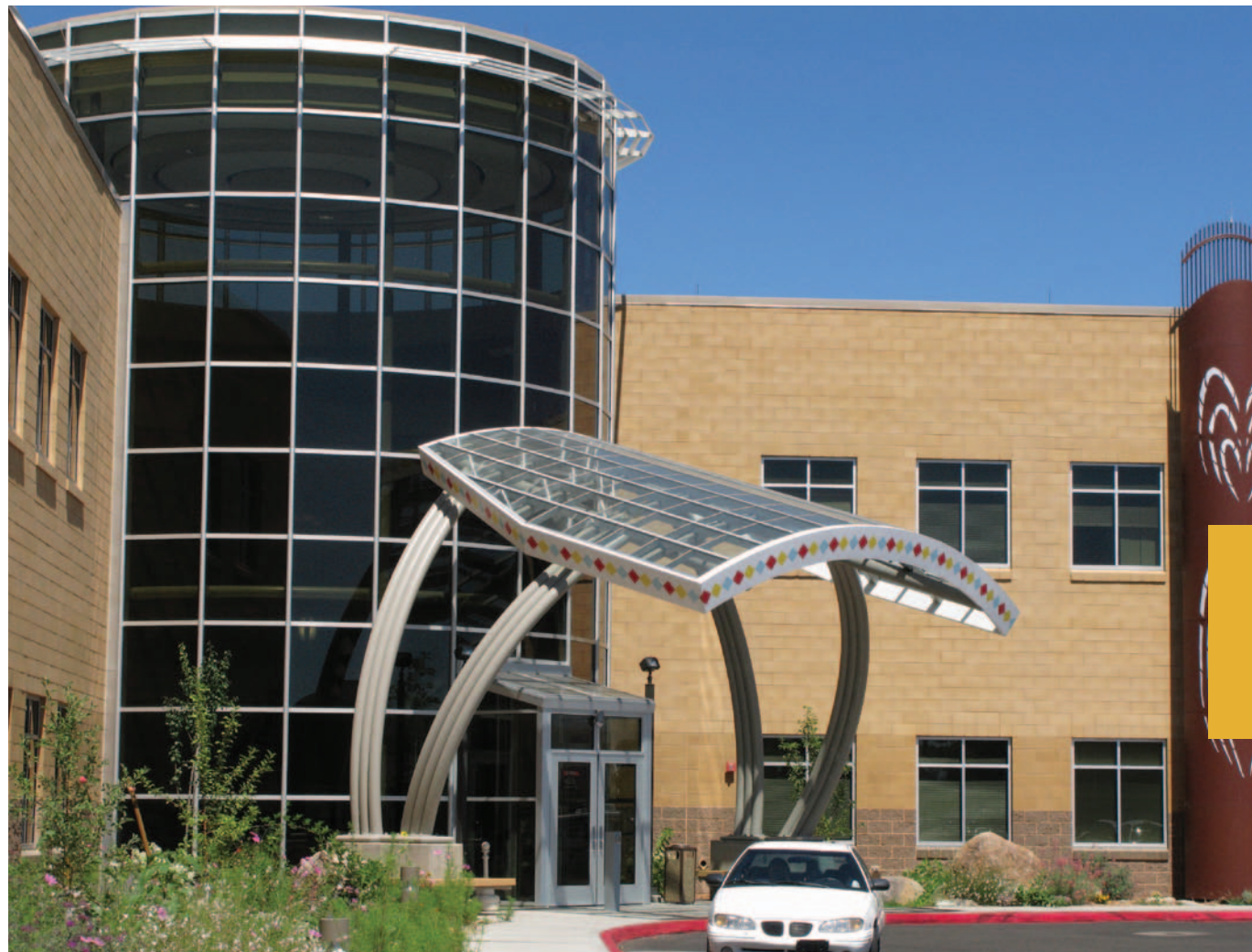
Brownfields redevelopment helped finance the new Tribal Health Center at the Reno-Sparks Indian Colony, near Reno, Nev.
