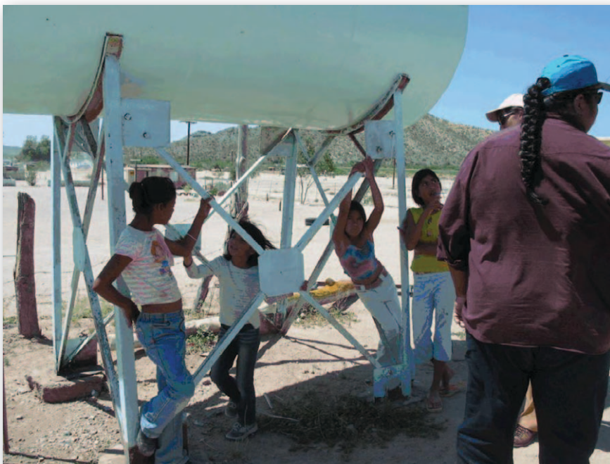
Water supply tank at the Quitovac Tohono O'odham Community in the U.S.-Mexico border region.
