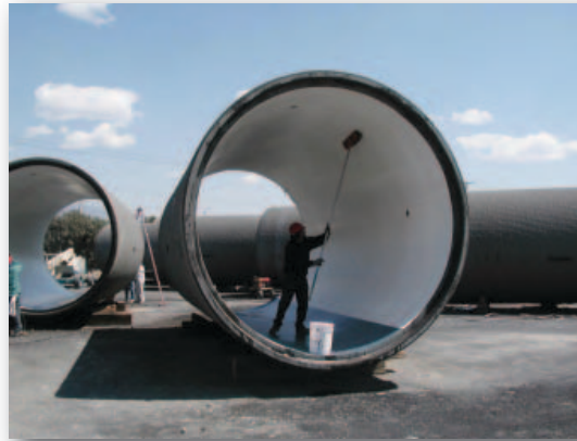
Preparing sections of new sewer pipe — part of Los Angeles’ effort to curb sewage spills.
