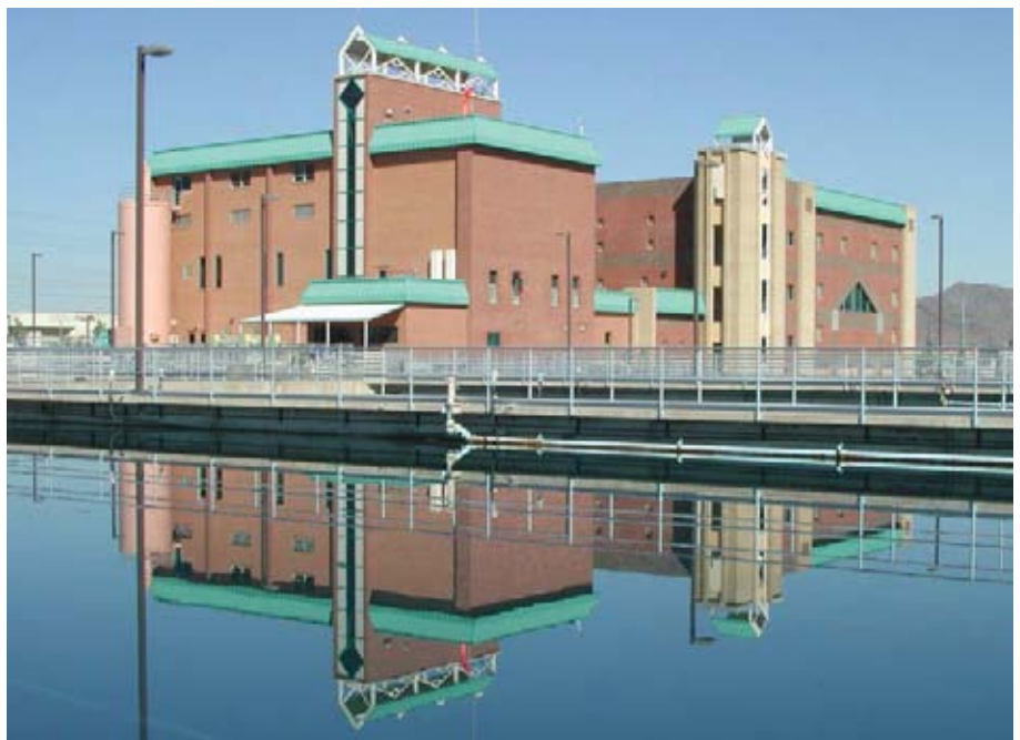
The Deer Valley Water Treatment Plant is one of Phoenix’s facilities for purifying drinking water.
