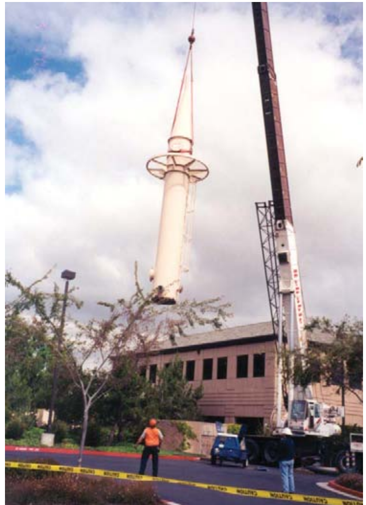
In Mountain View, Calif., responsible parties removed equipment that had treated TCE-contaminated groundwater by air-stripping, and replaced it with systems that release no TCE into the air.
