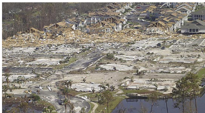
Gulfport, Miss. (Sept. 1, 2005) – The family housing area onboard Naval Construction Battalion Center Gulfport, Miss., shows considerable damage from Hurricane Katrina. U.S. Navy photo.
