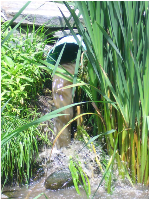
Figure 17: Discharge from Rushmore/Brigadoon Estates WWTP
