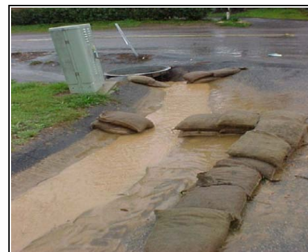
Poorly maintained BMPs can result in significant quantities of sediment being discharged to storm drains.
