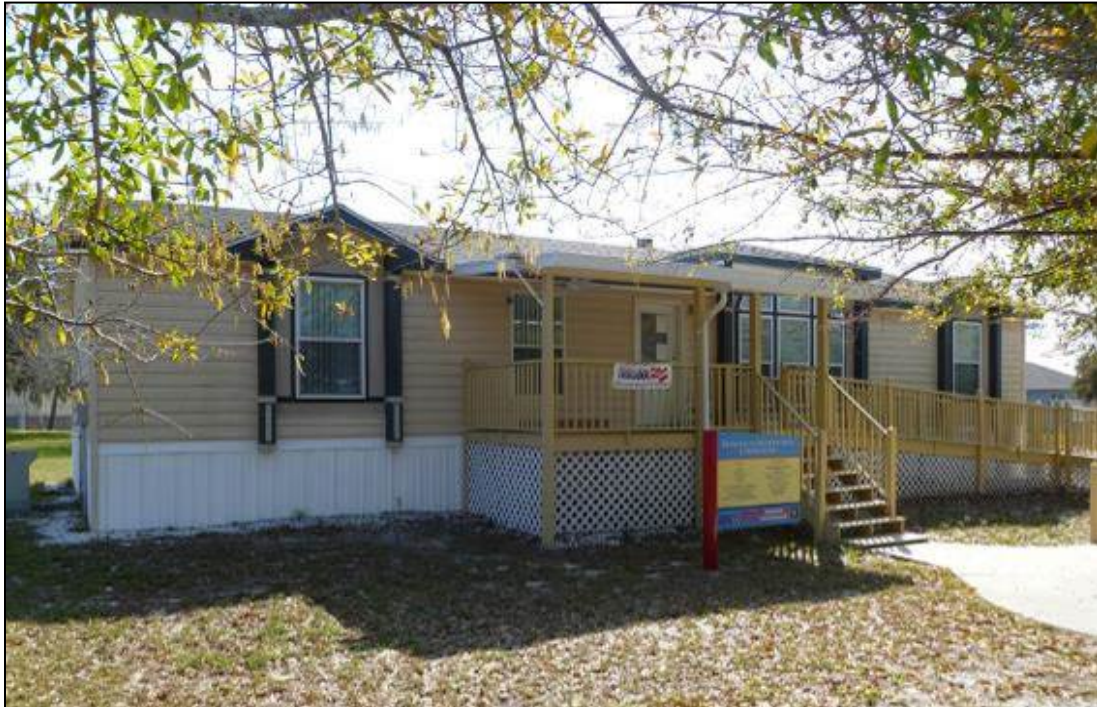
Figure 1. Florida Solar Energy Center MH Lab view of north exterior side
