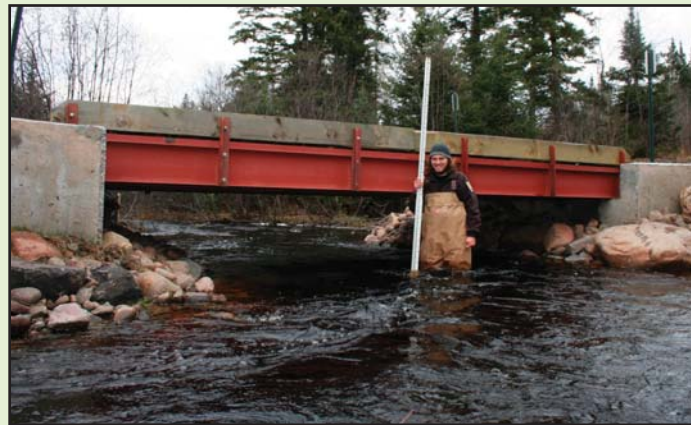
Above: The new free span bridge was built by the Iron County Forestry Department. This view is looking downstream. U.S. Fish and Wildlife Service student employee, Tyler Martin, is as happy as the fish. Service photo.
