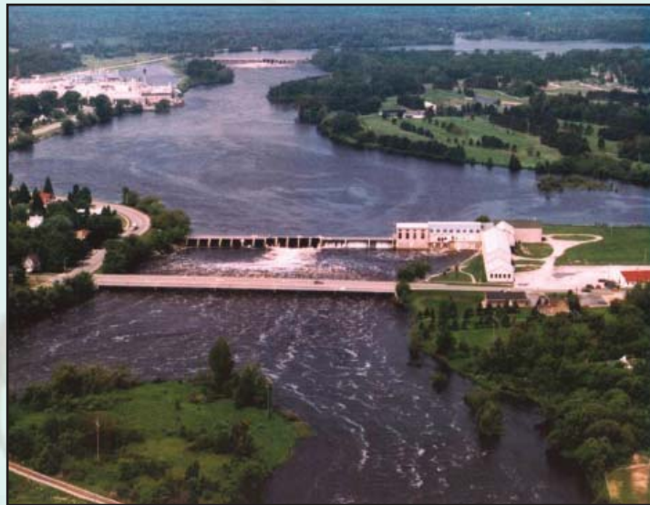
Below: North American Hydro's Menominee River Dam is part of the fish passage project. Service photo.
