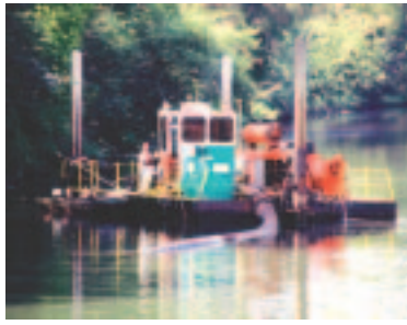
Figure 5. Hydraulic dredge on a river in Indiana.
