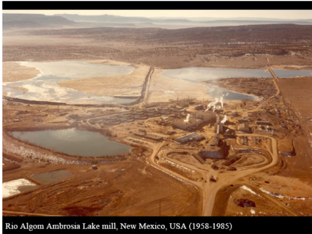
Rio Algom Ambrosia Lake mill, New Mexico, USA (1958-1985)
