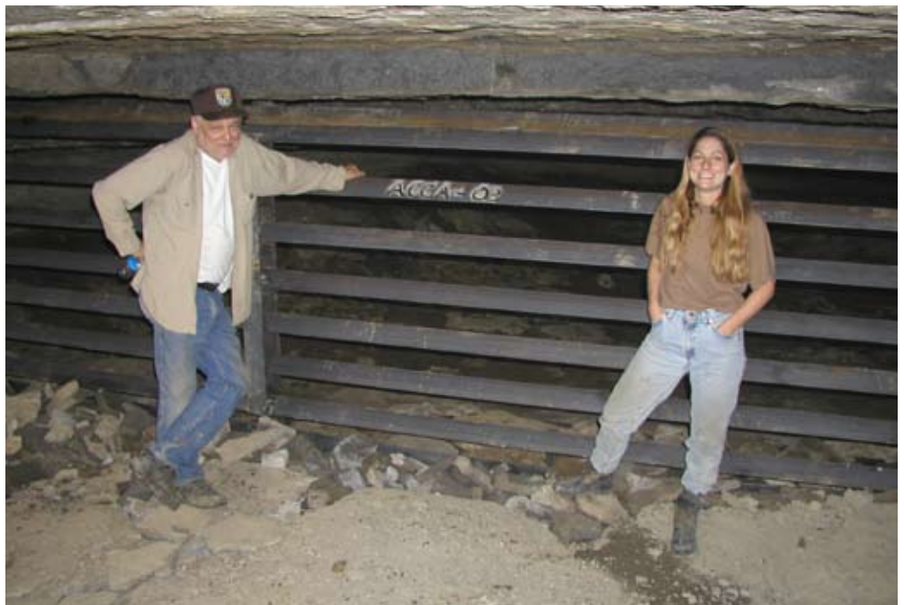
Gate designers Roy Powers and Kristen Bobo in front of the completed gate. Brent Harrel, USFWS photo
