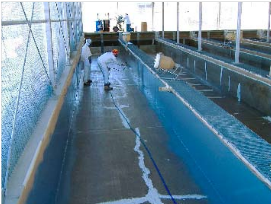
Contractors applying an environmentally safe coating in an LCT runway at Lahontan NFH.
