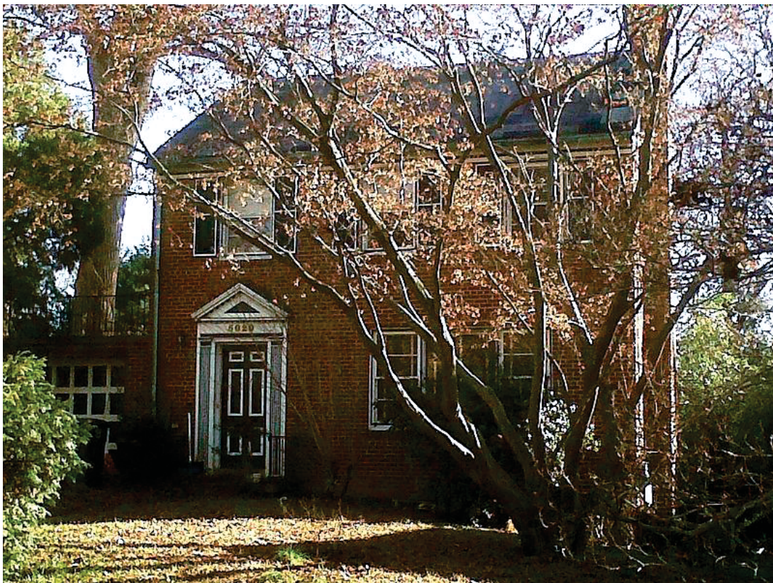
Figure 6: The Dr. Franklin E. Kameny House, Washington, DC. Photo by Farragutful, 2011. 43
