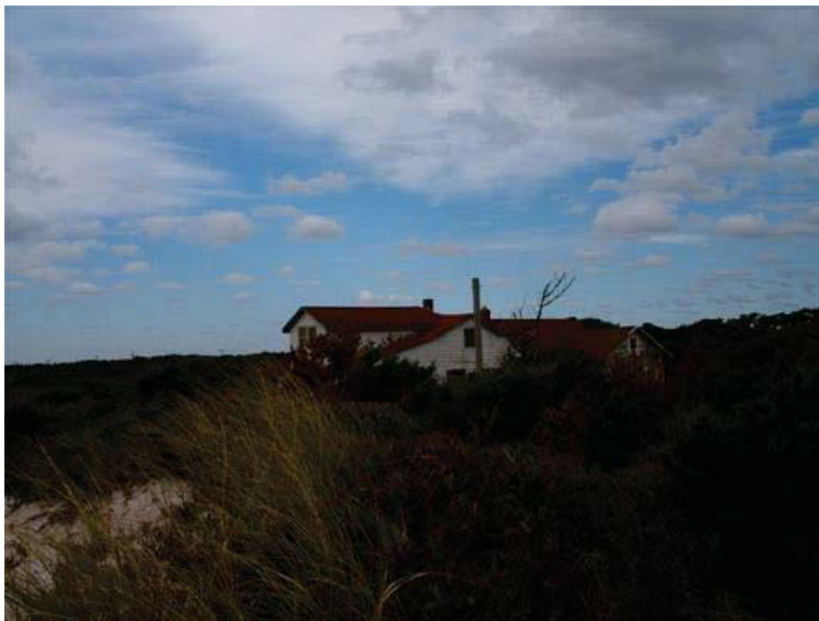
Figure 7: Carrington House, Cherry Grove, New York. Photo courtesy the National Park Service.
