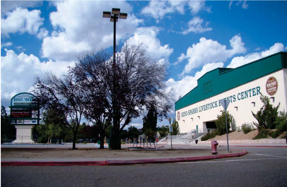
Figure 10: Washoe County Fairgrounds, July 2015. Photo courtesy of Nicholas-Martin Kearney.
