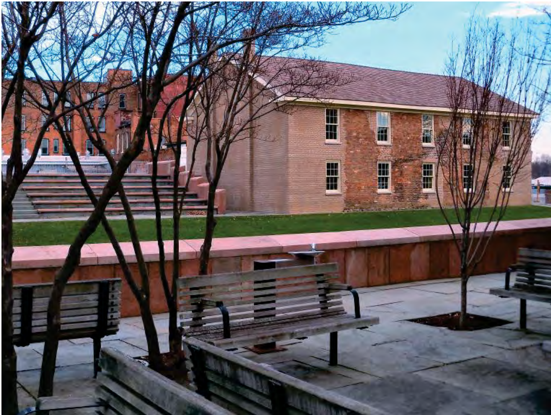
Figure 1: Wesleyan Chapel, 126 Fall Street, Seneca Falls, New York, site of the First Women's Rights Convention in the United States, 1848. The Chapel was listed on the NRHP on August 29, 1980. It is part of Women's Rights National Historical Park, established December 28, 1980. Photo by the author, 2011.
