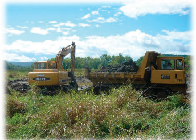
Figure 6: Wetland restoration work at Sudbury Wetland
