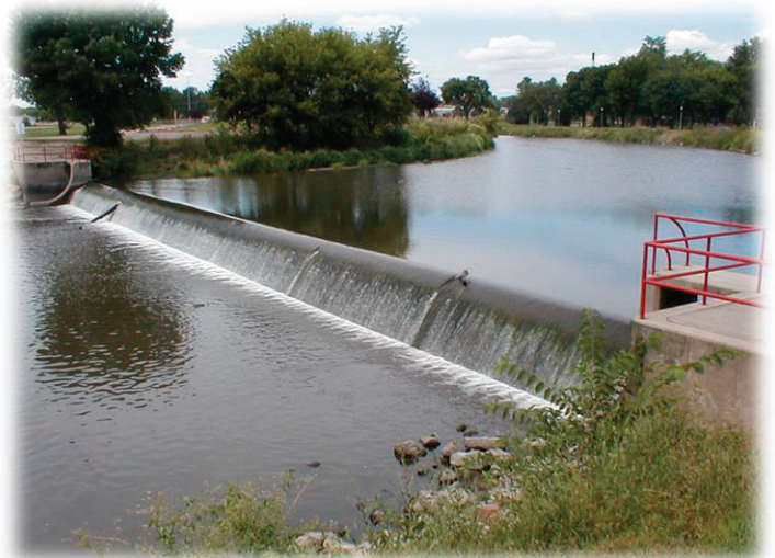
Figure 14: Luverne Dam prior to removal
