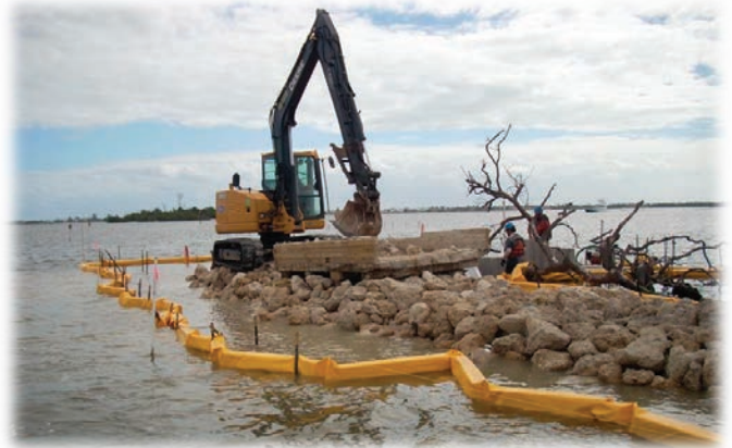
Figure 21: Wave break installation at Bird Island
