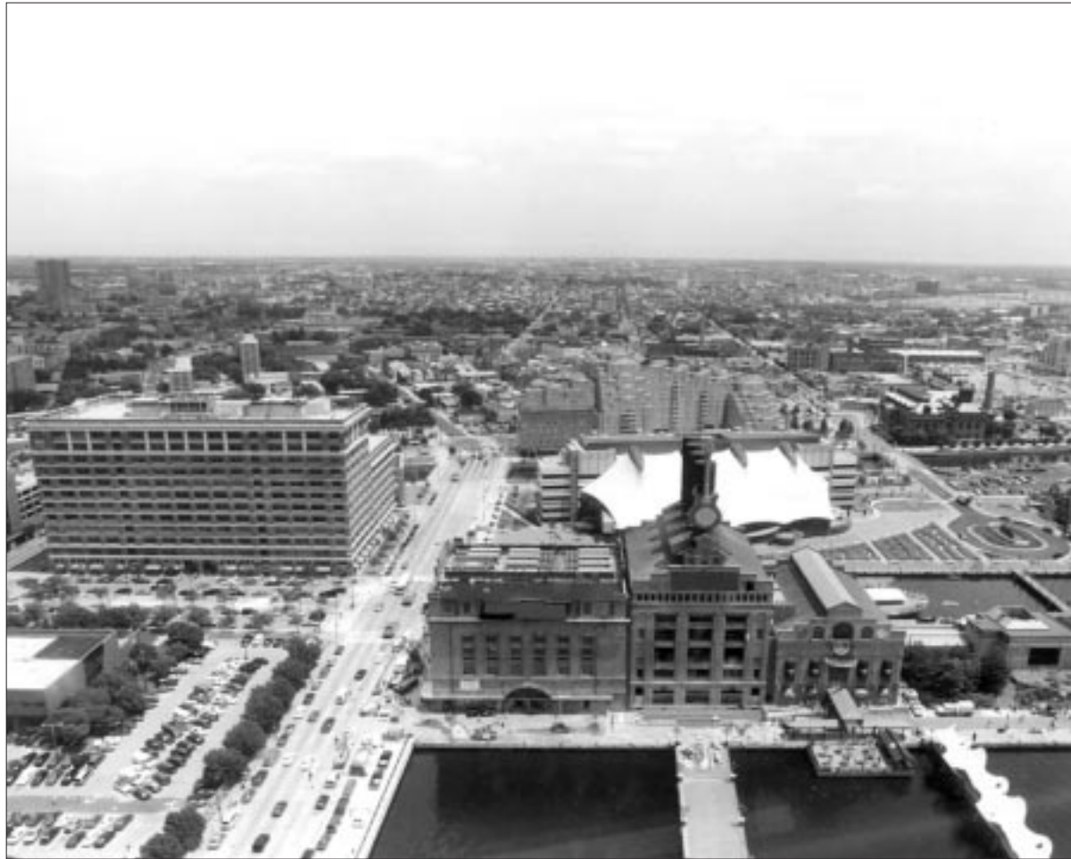
Office buildings, industries, residences, and transport systems, Baltimore, Maryland; east view from the Inner Harbor. Source: U.S. Department of Energy.
