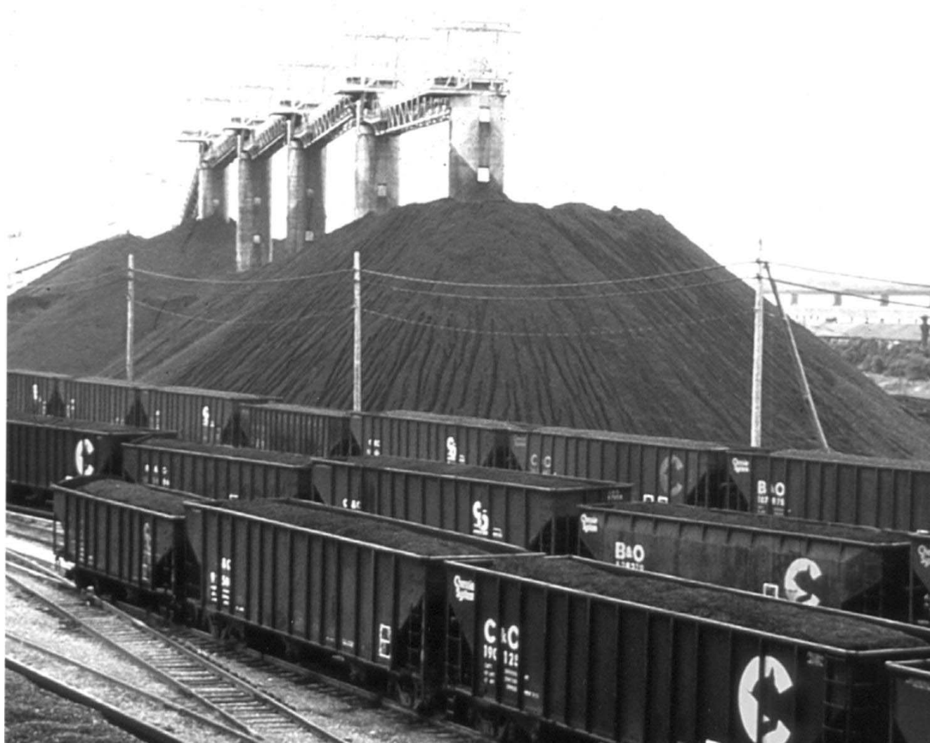
Coal yard, Curtis Bay, Maryland. Source: U.S. Department of Energy.
