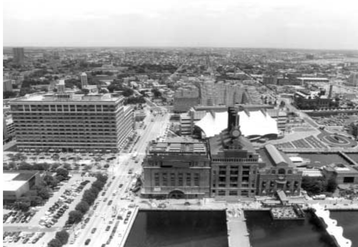
Office buildings, industries, residences, and transport systems, Baltimore, Maryland; east view from the Inner Harbor. Source: U.S. Department of Energy.
