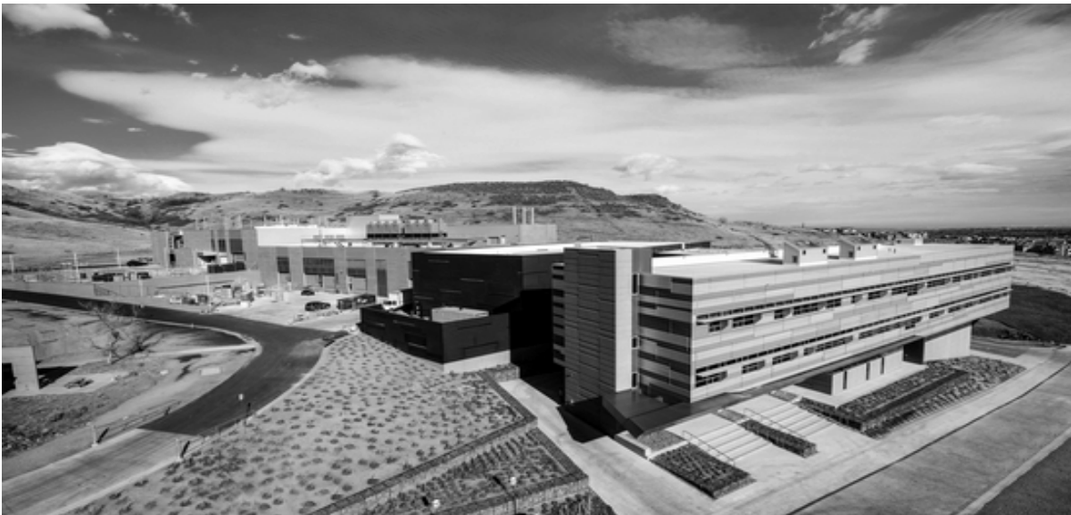
Figure 1. The Energy Systems Integration Facility at the National Renewable Energy Laboratory
