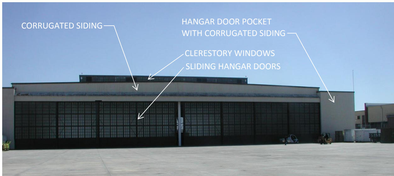
Figure 19. Typical building elements at east and west ends of aircraft bays (Mr. Richard Simonton, 2013).
