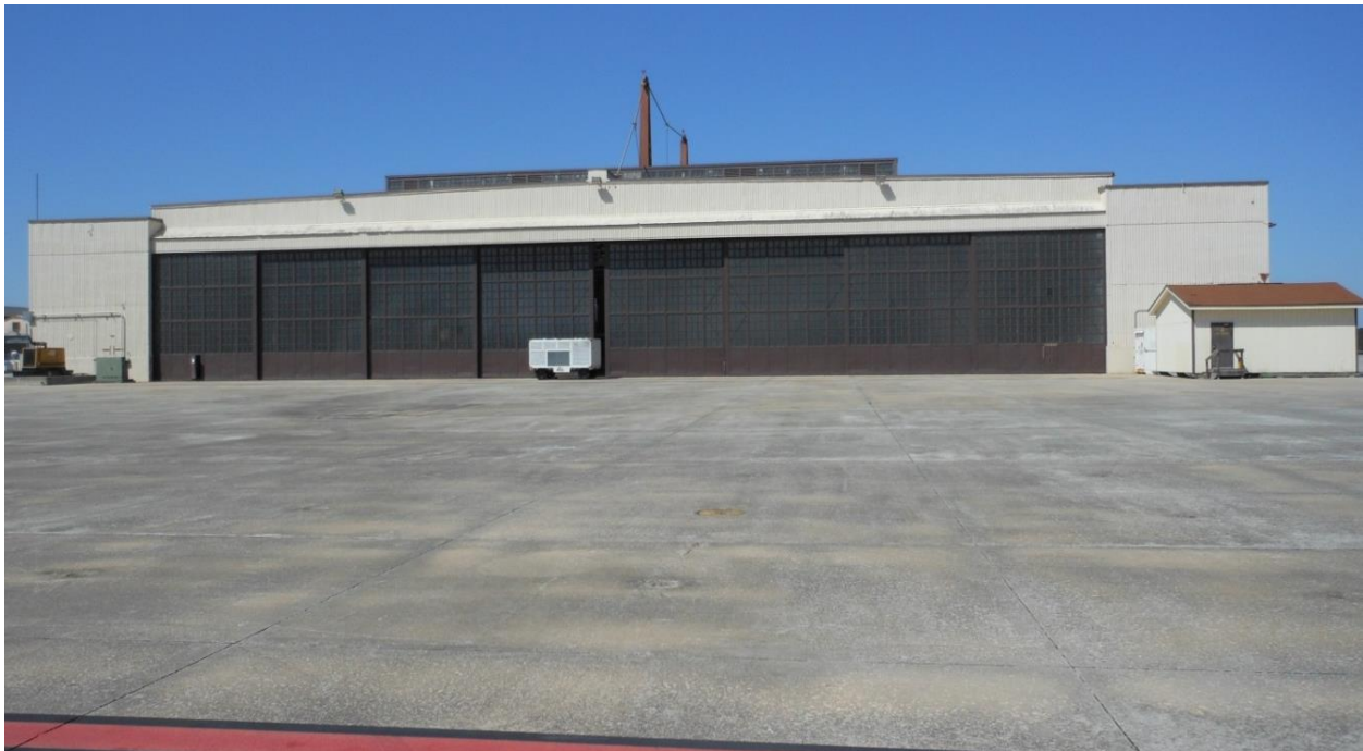
Figure 3. Landplane Hangar (1940), 114, 8DU11724, designed by Albert Kahn with modifications made at a later date, is a contributing element to the Landplane Hangar Historic District at NAS JAX. It is designated a Maintenance Hangar in the Florida Master Site Files. Note, a 300-foot apron lies between Hangars 114 and 115 (Ms. Kelly Nolte, 2013).
