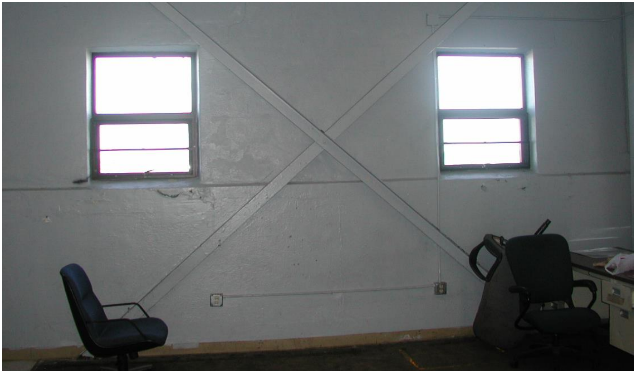
Figure 18. Typical replacement windows on north and south elevations (Mr. Richard Simonton, 2013).
