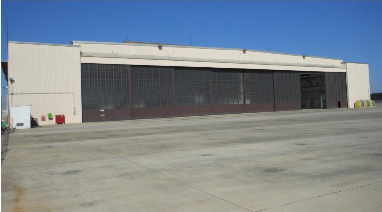
Figure 2. Landplane Hangar (1940), 113, 8DU11723, designed by Albert Kahn, is a contributing element to the Landplane Hangar Historic District, NAS JAX (Ms. Kelly Nolte, 2013).
