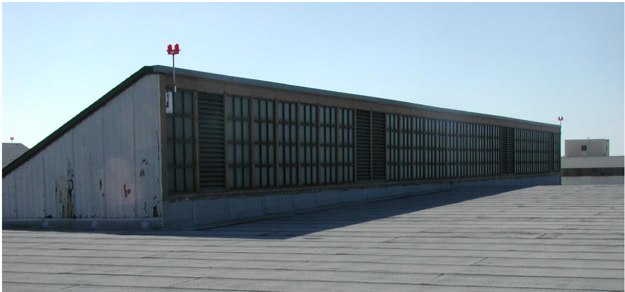
Figure 14. Typical rooftop sawtooth clerestory (Mr. Richard Simonton, 2013).
