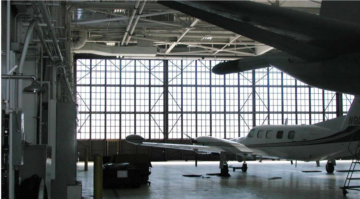
Figure 24. Interior view of hangar looking toward glazed hangar doors (Mr. Richard Simonton, 2013).
