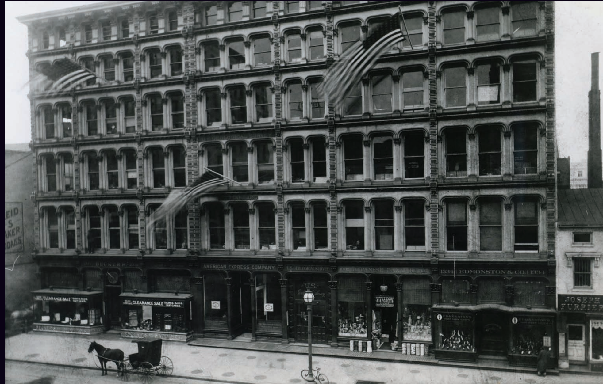
The Hooe Iron Building on F Street, NW housed the Solicitor General and one of the Assistant Attorneys General and his staff. When it was built in 1873, it was Washington's largest cast iron front structure. The building was razed in 1926. 16
