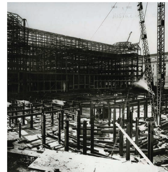
Looking southwest at the steel frame of the Department of Justice Building, December 1, 1932. The 10th Street side of the IRS building can be seen on the right. 27
