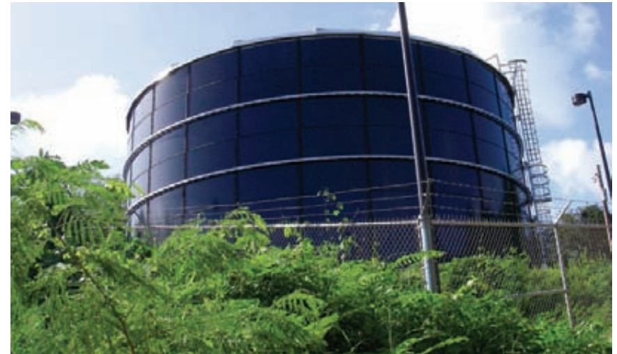
EPA provided nearly $3 million in grant funding to construct this one million gallon water storage tank and improve the distribution system in the Kannat Tabla area on the island of Saipan, in the Commonwealth of the Northern Mariana Islands (CNMI). The new tank is part of a number of system improvements that will eventually lead to 24-hour water on Saipan.
