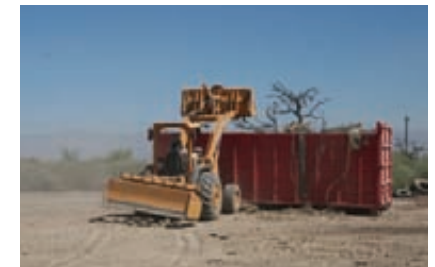
Road in Torres Martinez Reservation after cleanup.
