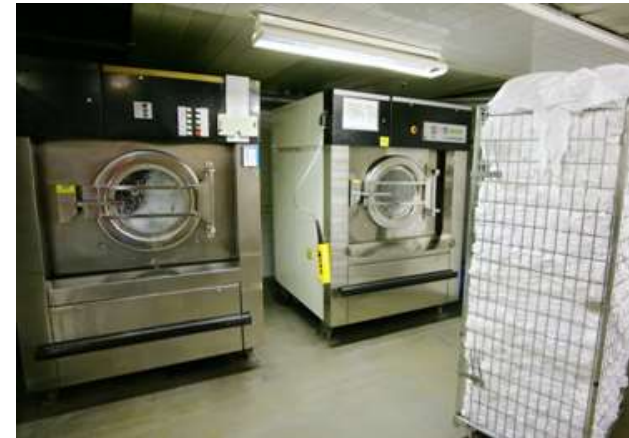
Washer Extractors 30 to 800 lbs/load 2-4 gallons of water/lb fabric
