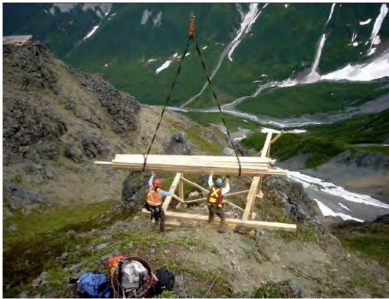
Photo 2-3. Slinging Decking Material for Drill Pad Construction
