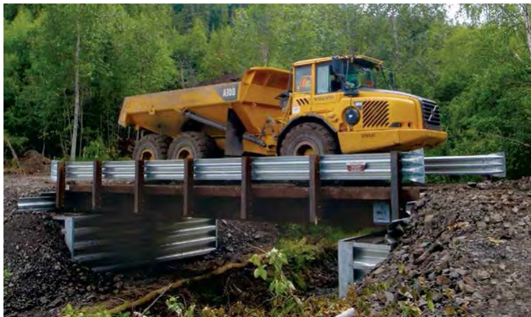
Photo 2-2. Example of Prefabricated, Modular Steel Vehicle Bridge
