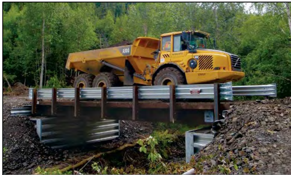
Plate 2.14: Example of a prefabricated modular steel vehicle bridge (Courtesy of Big R Bridge)
