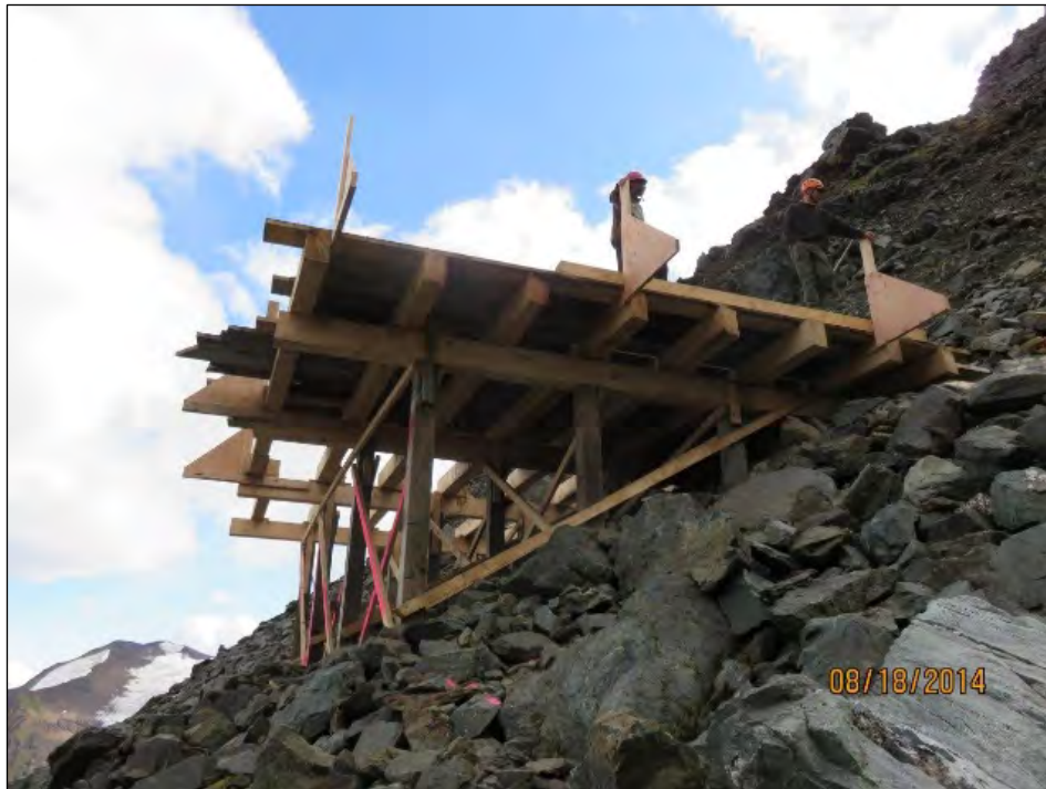
Plate 2.9: Final framing of pad
