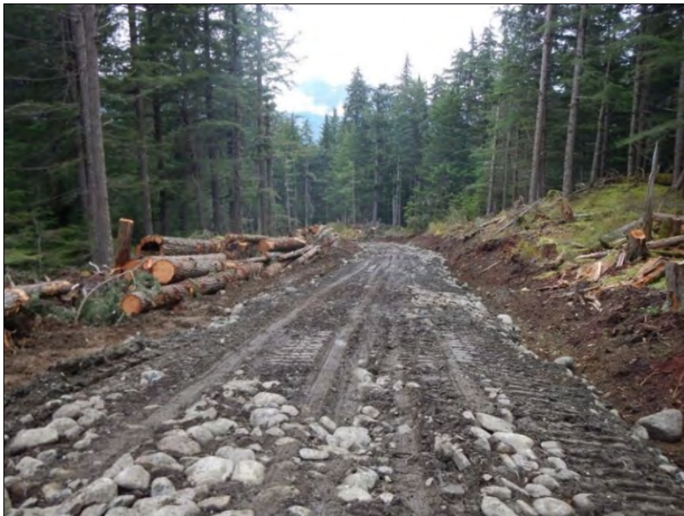
Plate 2.10: Construction of 2014 Exploration Access Road
