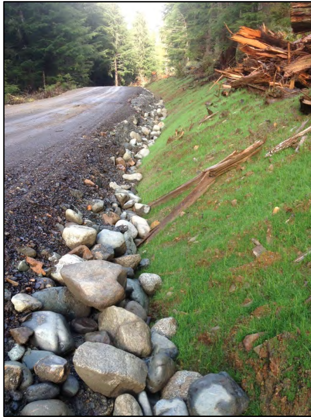
Plate 3.4: 2014 Exploration Access Road with Concurrent Reclamation
