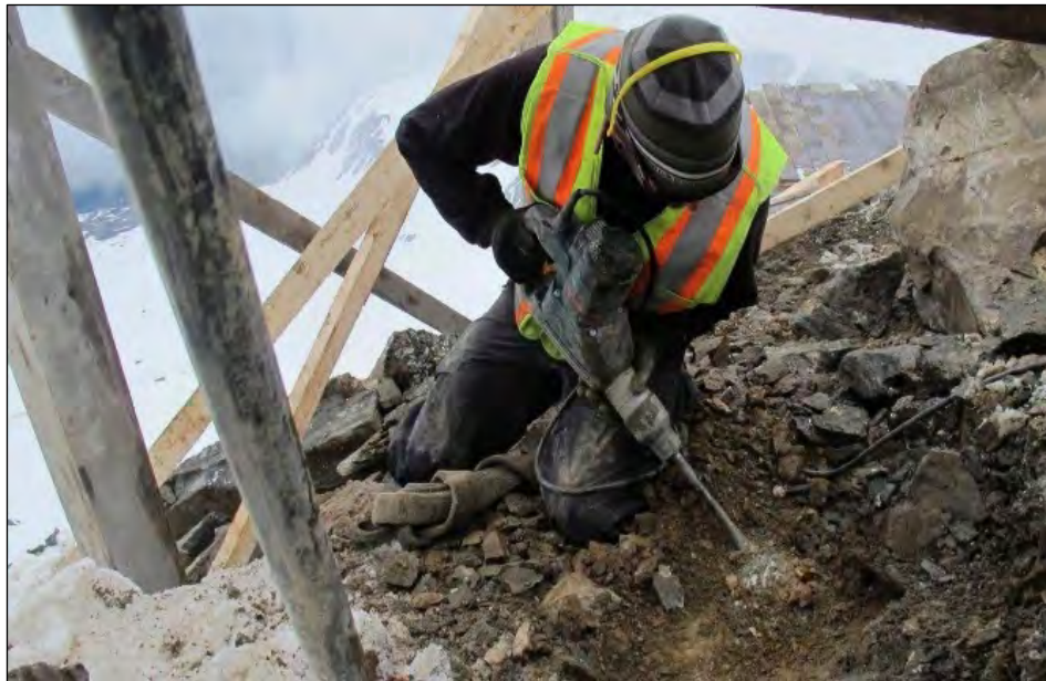
Plate 2.7: Setting of support timbers
