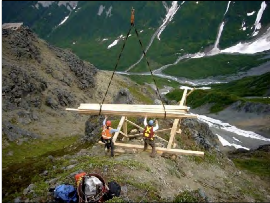
Plate 2.8: Slinging of decking material
