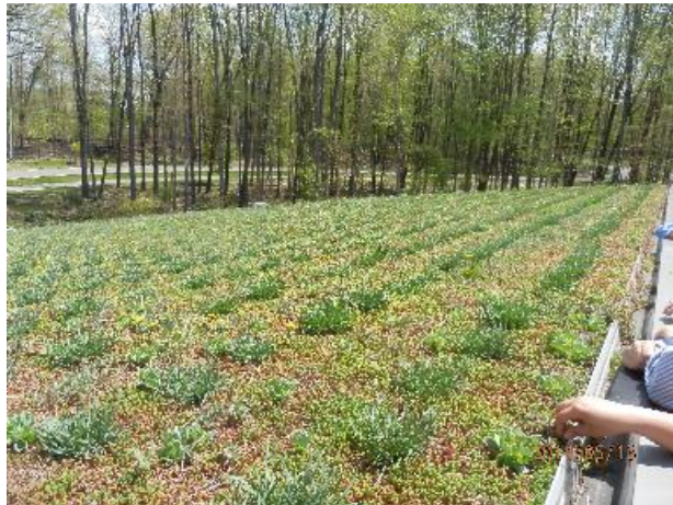
Green roof with adequate vegetation (Credit: EPA Region 5)
