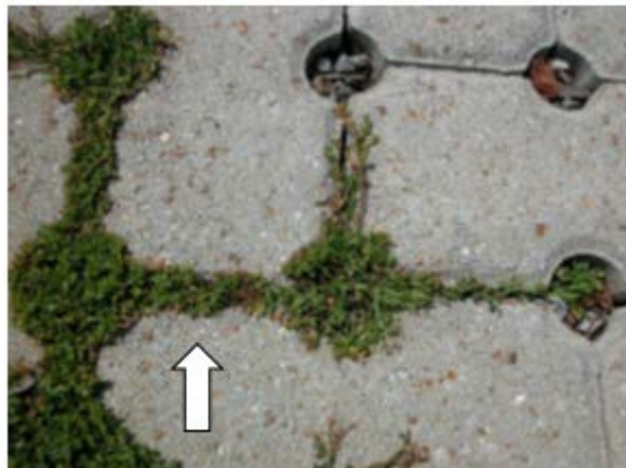
Photo 14-9. Weeds and moss between pavers may indicate a sediment problem. Herbicides should not be used on permeable pavement systems. (Credit: Bill Hunt, NCSU)
