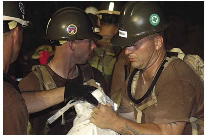
New Orleans (Sept. 24, 2005) - U.S. Navy Builder 1st Class Daniel McKee, right, assigned to Naval Mobile Construction Battalion Four Zero (NMCB-40), hands-off a sandbag to another Seabee while repairing a levee. A 150-foot sandbag wall was completed in time to beat the high tide, protecting Plaquemine Parish residents from any further damage caused by flooding as a result of Hurricane Rita. U.S. Navy photo.
