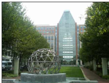
The James Madison Building at USPTO Headquarters
