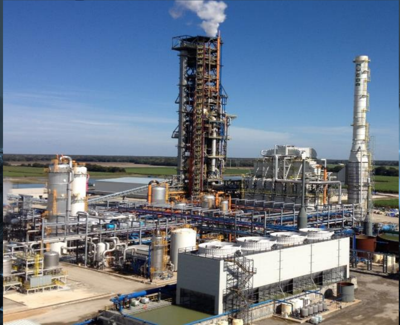
Photo: Nucor Steel Louisiana Energiron® DR plant
