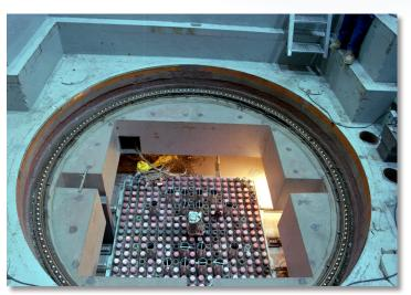
The TREAT facility operated from 1959 through 1994, when it was placed in safe-standby mode. A resurgence of the United States and international interest in developing innovative nuclear technologies has restored the demand for transient testing. INL's Resumption of Transient Testing Program (RTTP) is working to re-establish transient test capability and is on track to resume operations in FY 2018.
