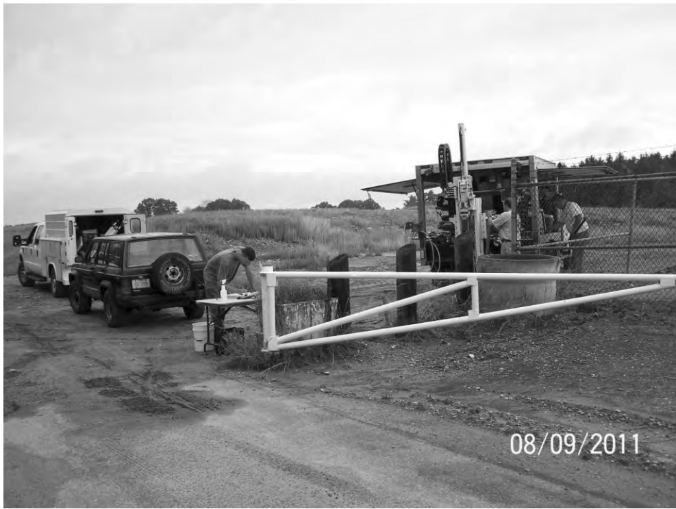
Photo 38: View looking northeast at boring location GP-1.
