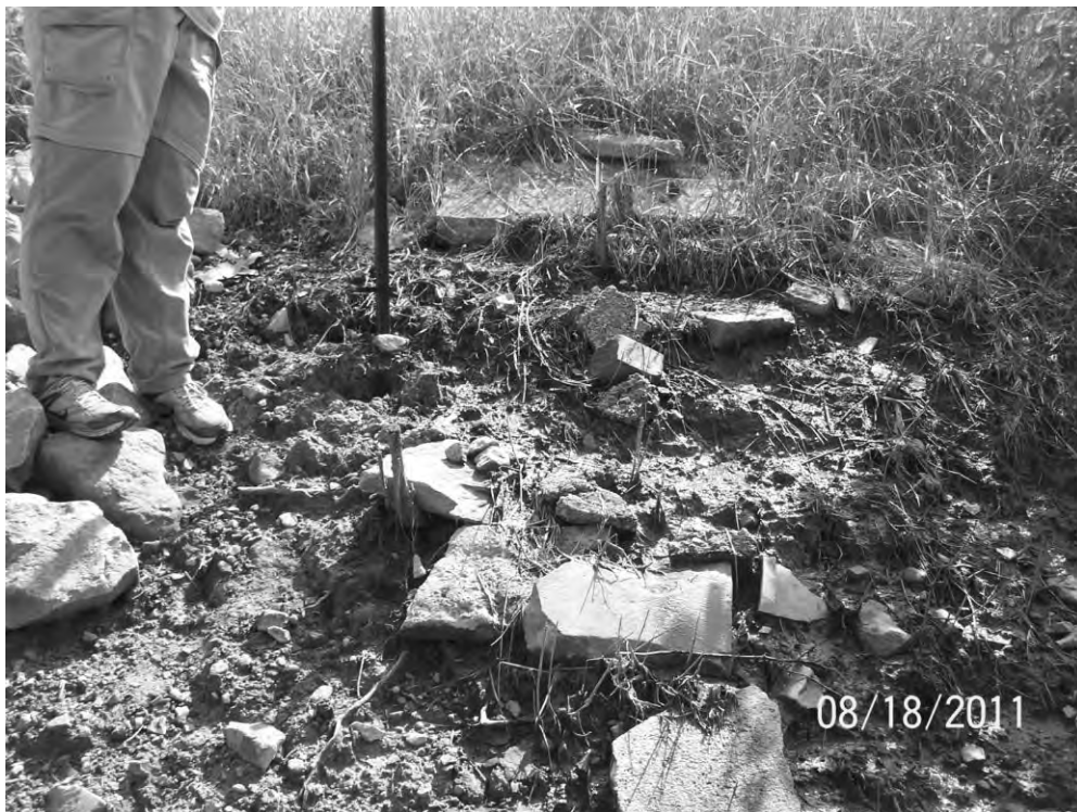
Photo 10: Leachate seep area halfway up bank of Raccoon Creek at southern edge of middle riprap area.
