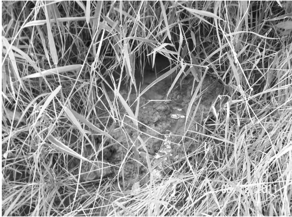
Photo 7: Leachate seep along Raccoon Creek just upstream of “S” curve.
