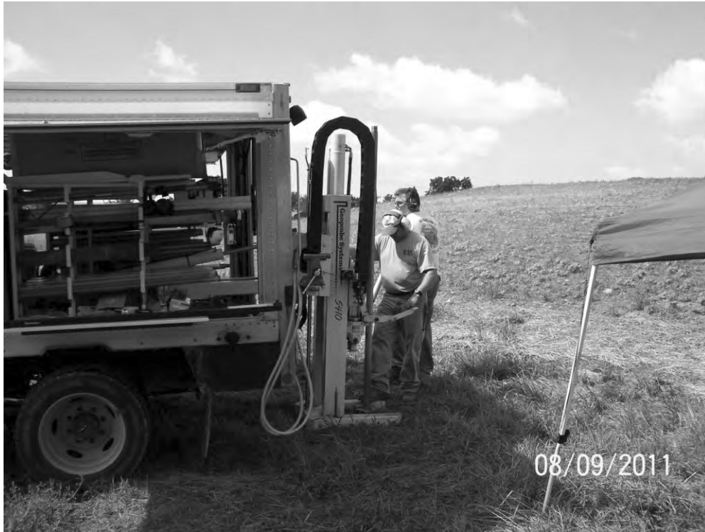
Photo 16: Boring operations at location GP-2 near southeast corner of fill.
