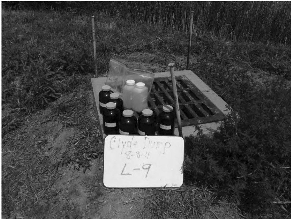
Photo 31: View looking east at leachate manhole and sample location L-9.
