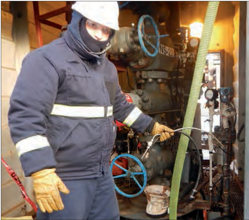
Soon after summer ends, BSEE's Alaska inspectors need to shield themselves from the elements. Because oil and gas production does not stop when the weather turns cold, BSEE's inspectors still need to visit Alaska's artificial Northstar Island, which lies in state waters, but has wells that extend to the federal OCS.
