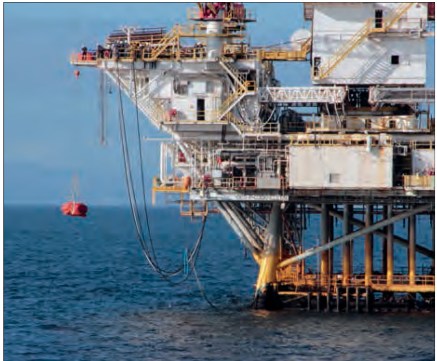
The size of loads lifted by offshore cranes can be substantial. The crew members seen in the upper left portion of this photograph provide a sense of scale. BSEE has been working with offshore operators to reduce the number of lifting incidents, which have ranged from 110 to 243 per year over the past decade.
