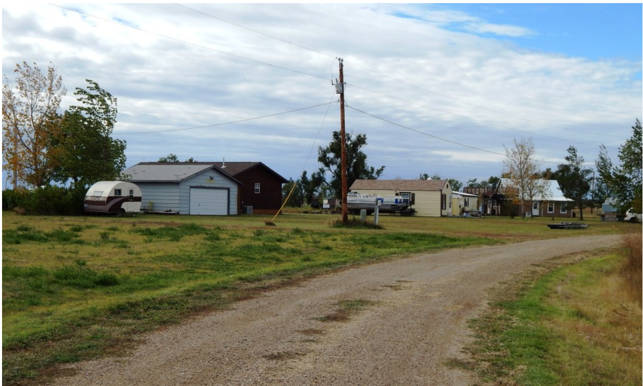
Looking southwest at an array of cabins located within Shadehill's West Cabin Area sites. The cabin sites are described in RECLAMATION records, from near to far, as sites W08, W09, and W10.
