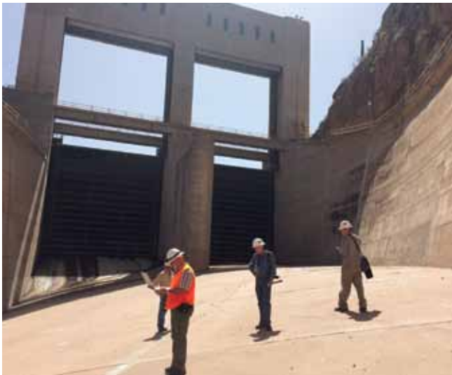
Inspections of Reclamation-owned facilities include extensive on-site examinations, as seen at Mormon Flat Dam on the Salt River in AZ.
