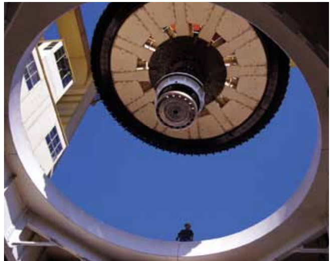
A worker observes a rotor being replaced at Davis Dam.
