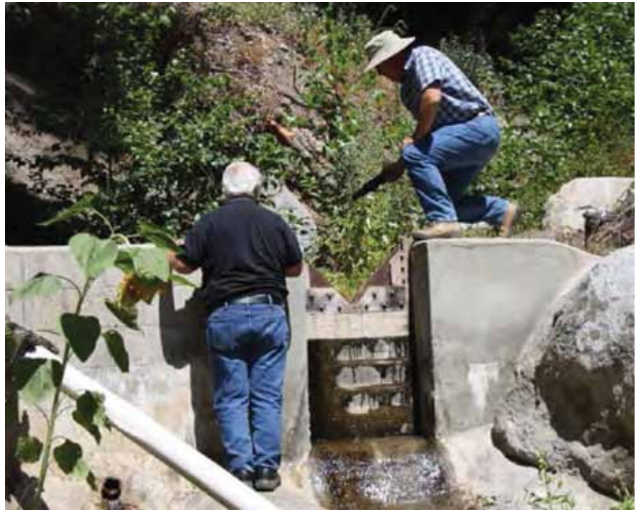
La Jolla Indian Tribe members examine a weir on their nearly 10,000-acre reservation in southern California. An emergency drought project funded by Reclamation successfully enhanced the Tribe's ability to collect surface water.
