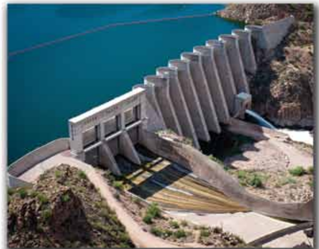
From top to bottom, Davis Dam (Colorado River, AZ/NV), Hoover Dam (Colorado River, AZ/NV) and Bartlett Dam (Verde River, AZ)
