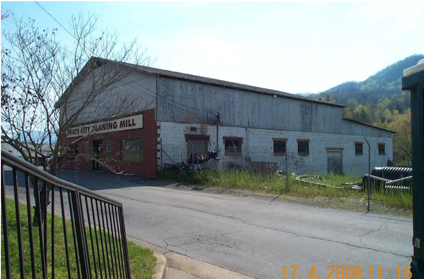
#20 Egan Construction, side view from opposite side of Water Street
