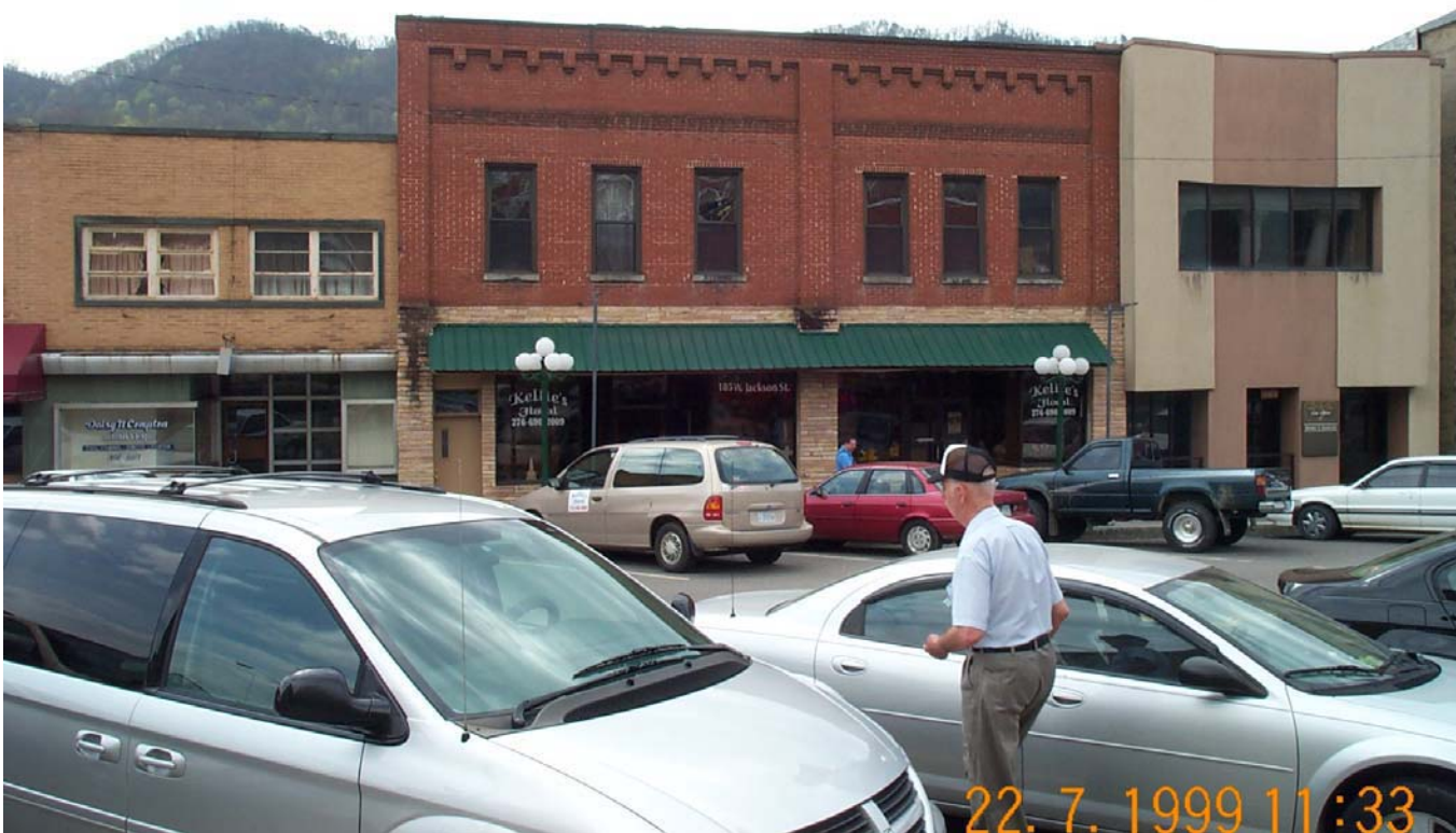
#10 Kelly's Floral and Gifts, front view from opposite side of Jackson Street (building w/ green roof)
