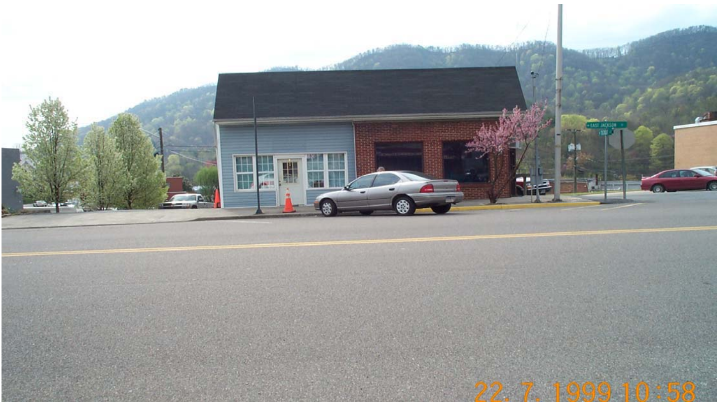
#2 East End Barber Shop/Vacant, front view from opposite side of Jackson Street
