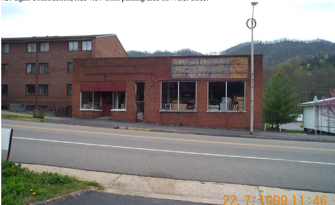
#21 Vacant/ Old Chapman Construction, front view from opposite side of Jackson Street
