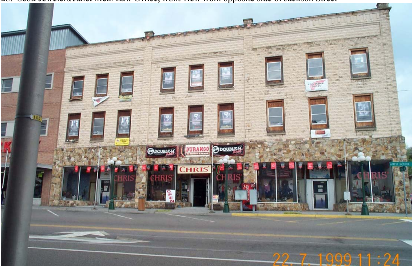
29. Chris' Department Store, front view from opposite side of Jackson Street
