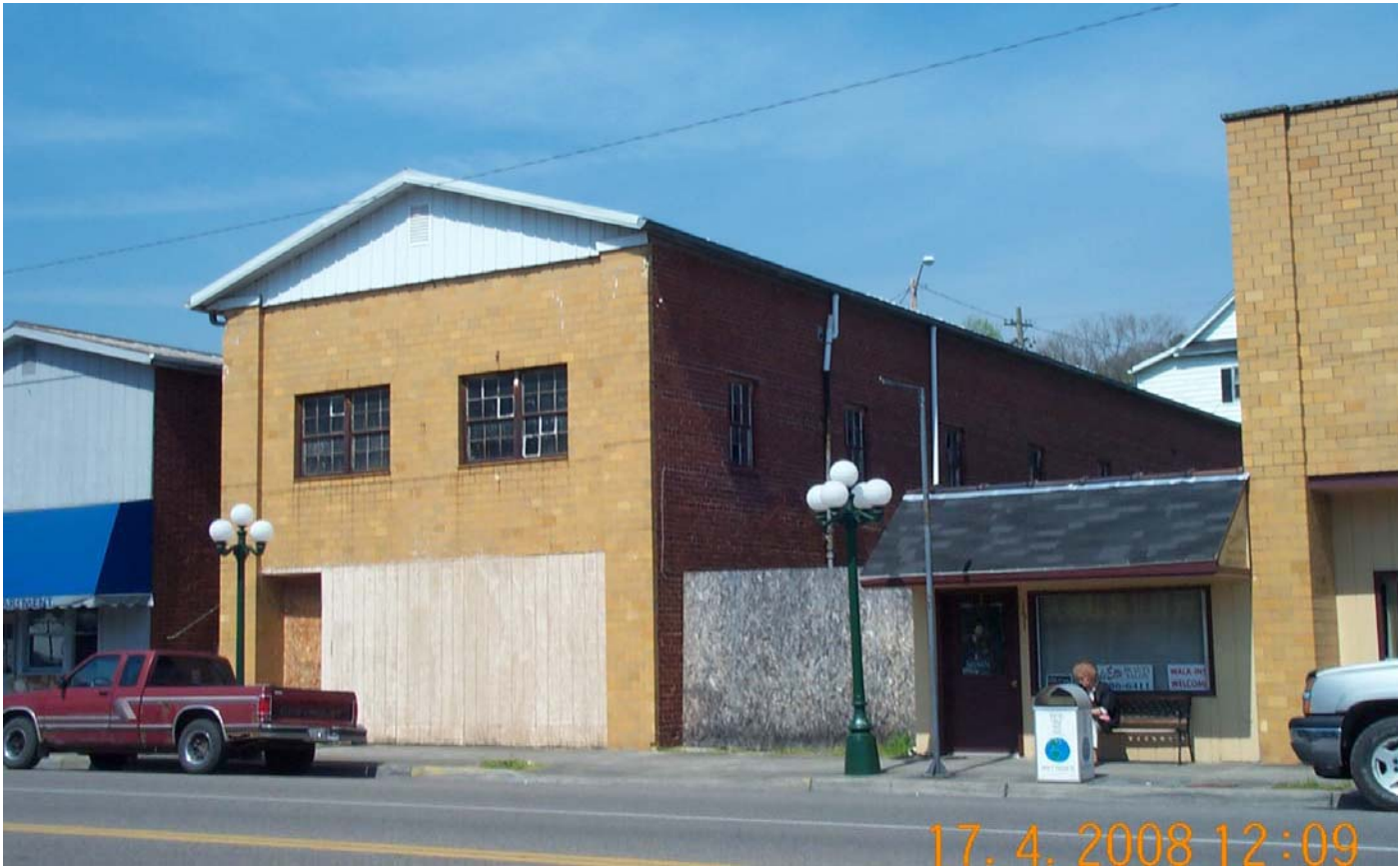
#31 Vacant/Old ABC Store, front and side view from opposite side of Jackson Street
