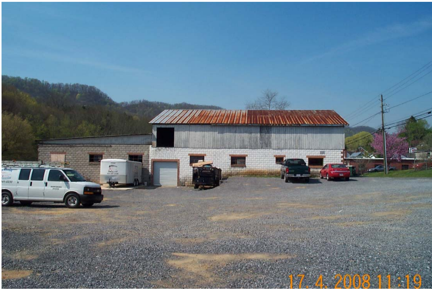
#20 Egan Construction, side view from parking area on Water Street
