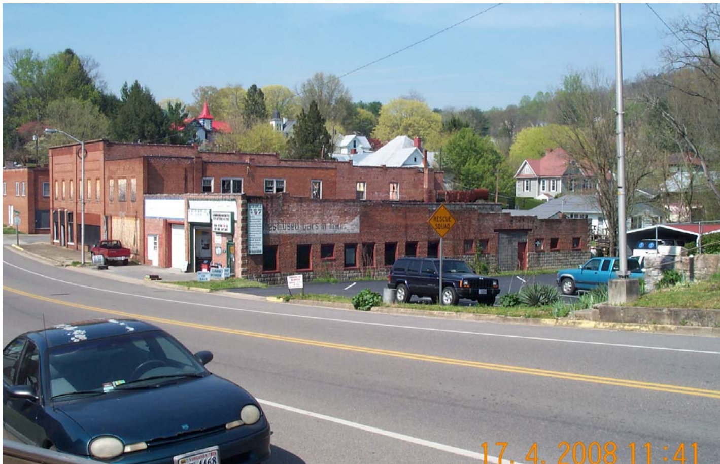
#24 Battery Depot, side view from opposite side of Jackson Street
