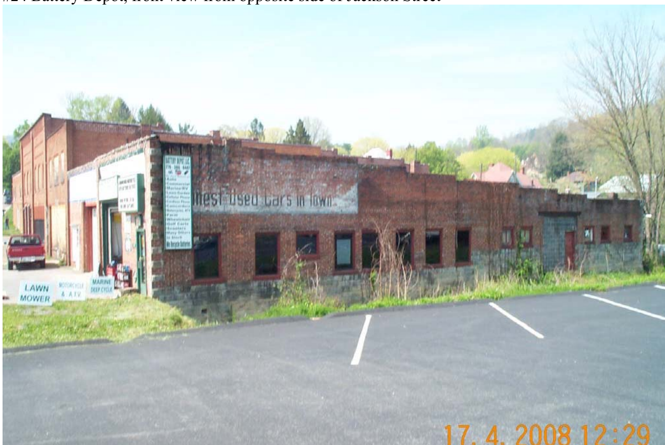
#24 Battery Depot, side view from parking Lot, Jackson Street
