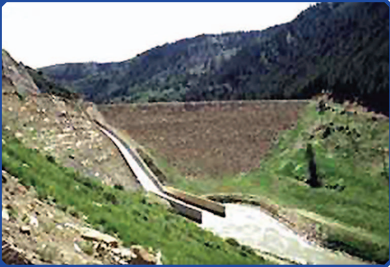
Downstream face of Paonia Dam, Colorado.
