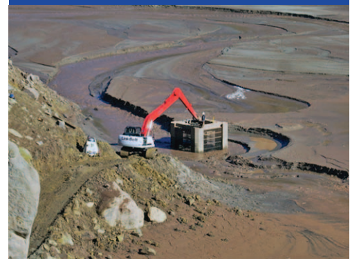
Long-reach excavator removing sediment and debris from around the intake tower at Paonia Reservoir, Colorado, in November 2014 (see the 2014 photograph on previous page of the manual clearing process by hand).
