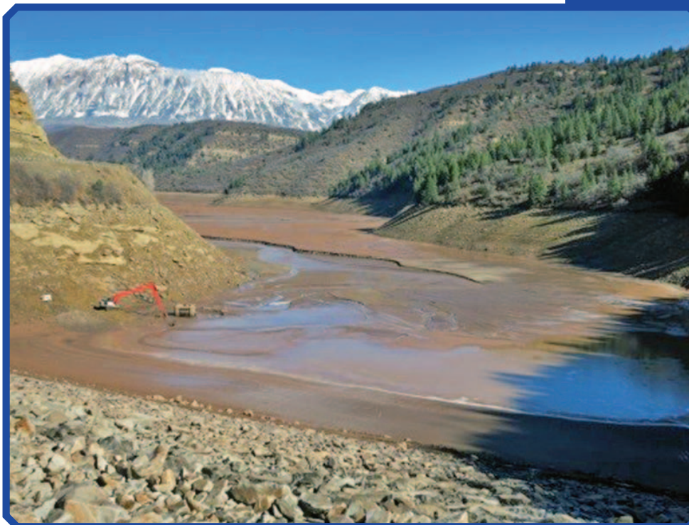
Long-reach excavator removing sediment and debris from around the intake tower at Paonia Reservoir, Colorado, in November 2014 (see the 2014 photograph on previous page of the manual clearing process by hand).
