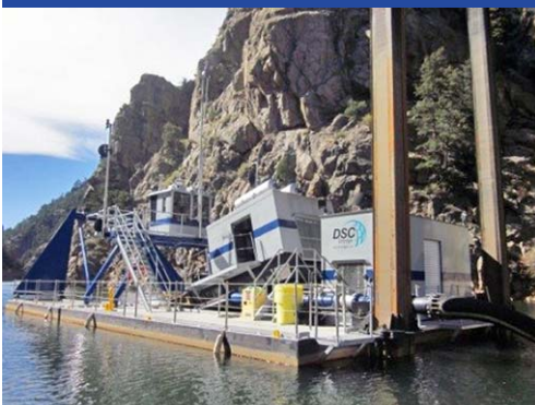
Dredging at Strontia Springs Reservoir, Colorado. Photograph by Tim Randle.
