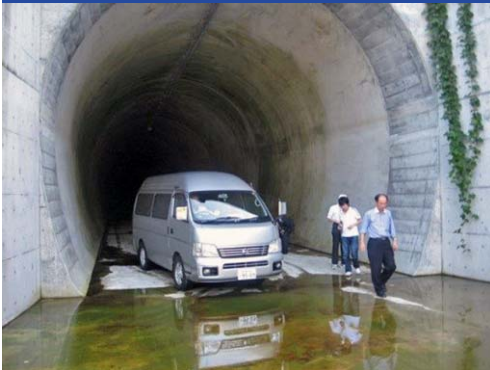
Sediment bypass tunnel at Miwa Dam, Japan. Photograph by Tim Randle.
