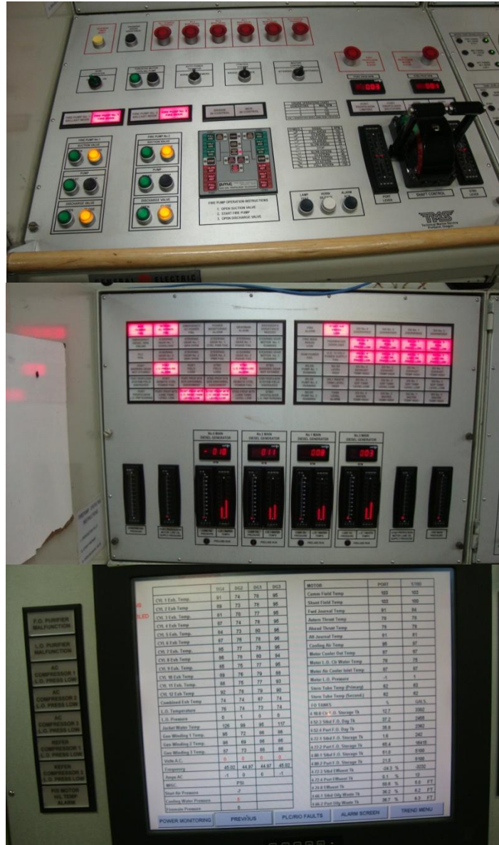
Figure 7. Engine Room Machinery Control Station
