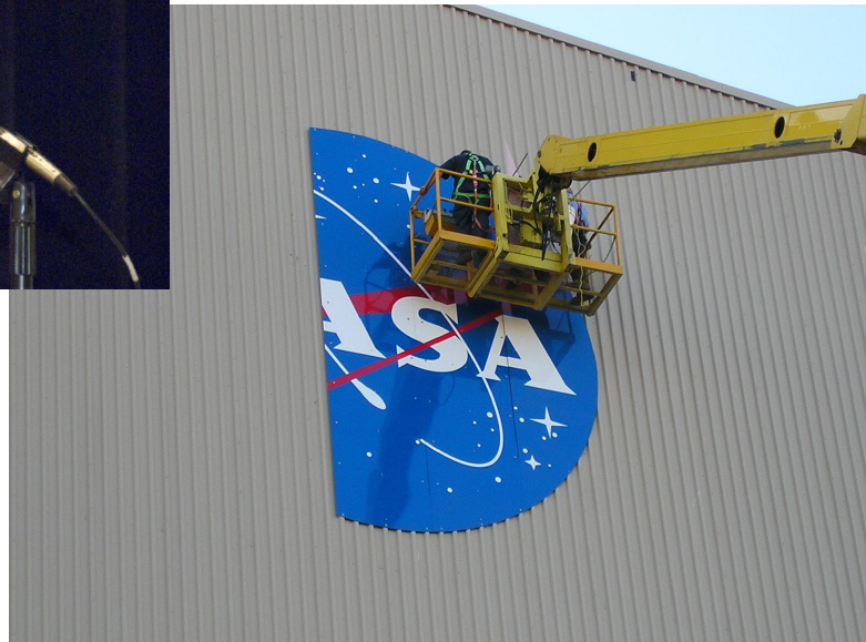
Figure 66: Installation of the NASA meat-ball on the new facility.
