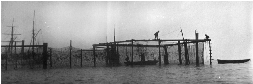
Salmon trap at Pt. Roberts, Wash., inspected by staff of the Albatross in 1895, courtesy of the National Archives.
