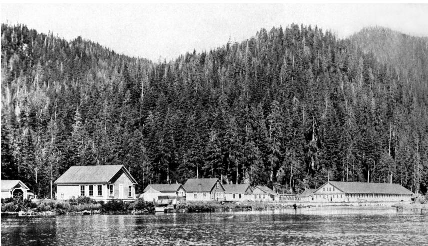
Yes Bay, Alaska, hatchery buildings (Jones, 1914).
