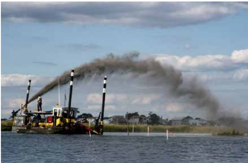
Salt marsh restoration in Jamaica Bay has tried a variety of experimental techniques to increase marsh elevation, including spraying the marsh surface using a swing-ladder dredge. Image credit: USACE New York District.
