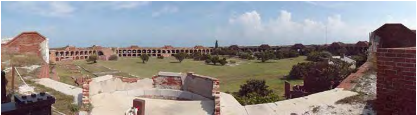
Historic Fort Jefferson is a six-sided structure built on a landform that is impacted by coastal processes. Image credit: Marcy Rockman, NPS.
