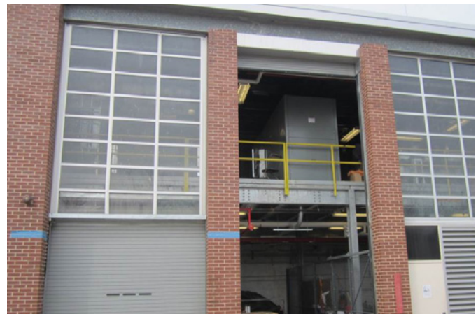
Figure 9.5. Photo of elevated platform in maintenance building on Liberty Island.
