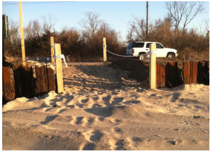
Figure 9.8. Photos of Aviation road bulkhead (left) and area where section was removed (right). Note: Planned removal of the Aviation road bulkhead to allow shoreline migration was delayed and only a section was removed initially for safe access. Removal of the bulkhead is now proceeding.
