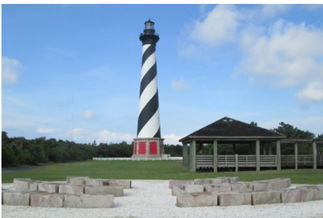
Figure 5.3. After multiple hard stabilization protection efforts proved unsuccessful, the Cape Hatteras lighthouse at Cape Hatteras National Seashore, North Carolina, was moved inland from the eroding beach using a railway in 1999. Photograph by NPS.
