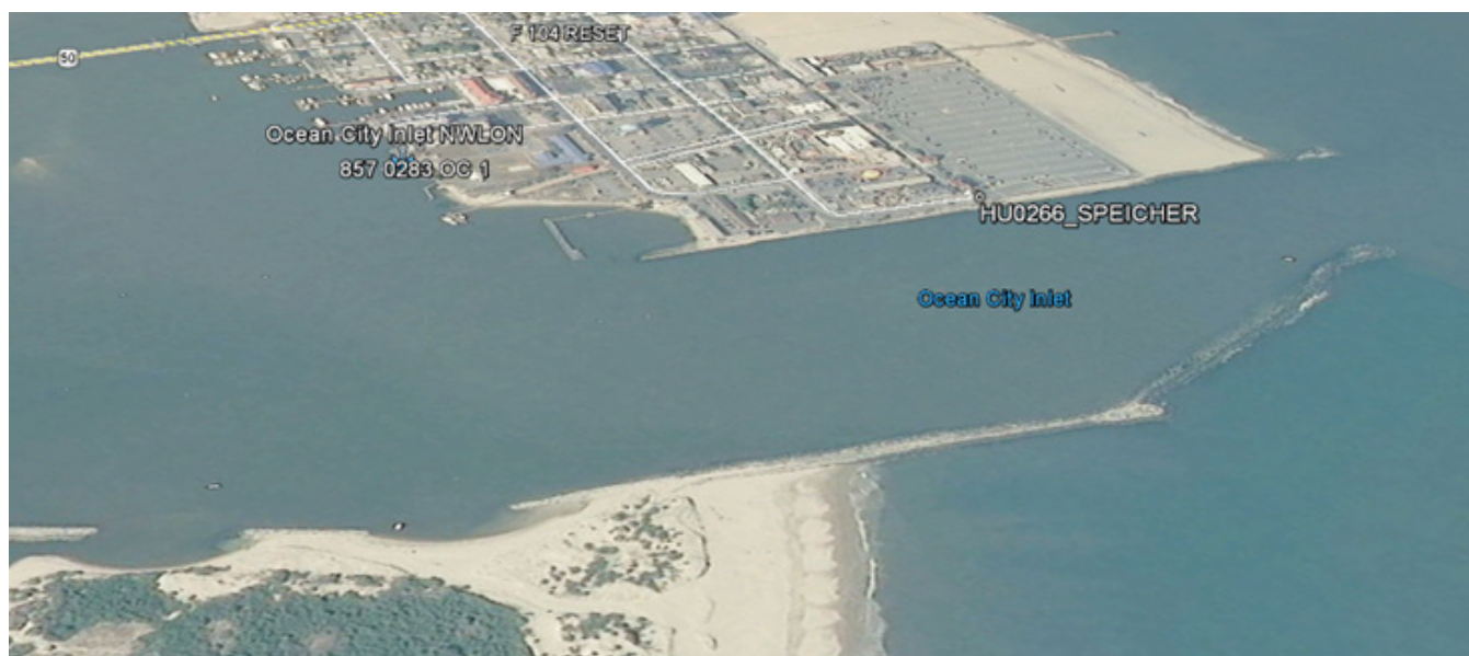
Figure 8.4. Ocean City Inlet jetty and breakwaters on the north end of Assateague Island National Seashore in 2011. Photograph by NPS.
