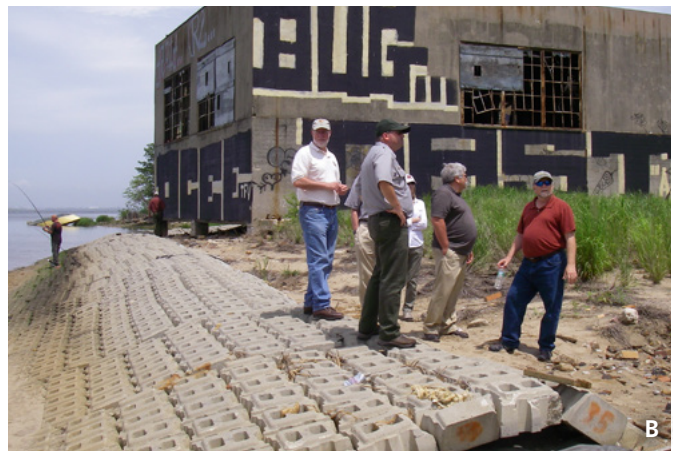
Figure 8.7. Examples of hybrid approaches to living shorelines. Notes: (a) This hybrid approach to a living shoreline uses natural and nature-based features by combining a planted marsh with a rock sill. Photograph from Bilcovic and Mitchell (2011). (b) The vegetation component of this hybrid approach at GATE was unsuccessful, leaving only shoreline armoring. Photograph by NPS.
