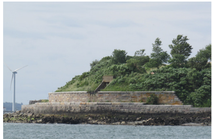
Figure 8.2. A seawall protects Fort Warren on Georges Island at Boston Harbor Islands National Recreation Area. Photograph by NPS.
