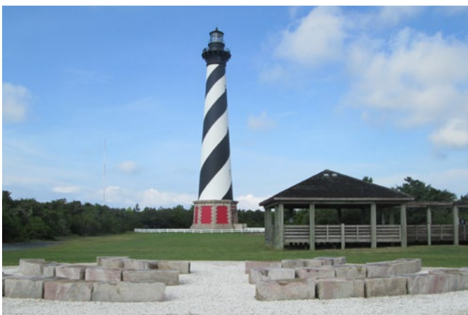
Figure 5.3. After multiple hard stabilization protection efforts proved unsuccessful, the Cape Hatteras lighthouse at Cape Hatteras National Seashore, North Carolina, was moved inland from the eroding beach using a railway in 1999. Photograph by NPS.
