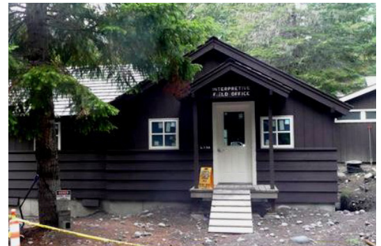
This historic Mt. Rainier office building is nearly identical to the original after Passive House renovations. A couple of subtle differences include the new concrete foundation with crawl space vents, and new energy-efficient casement windows.
